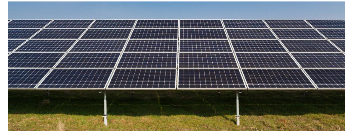
Fixed-tilt installation
