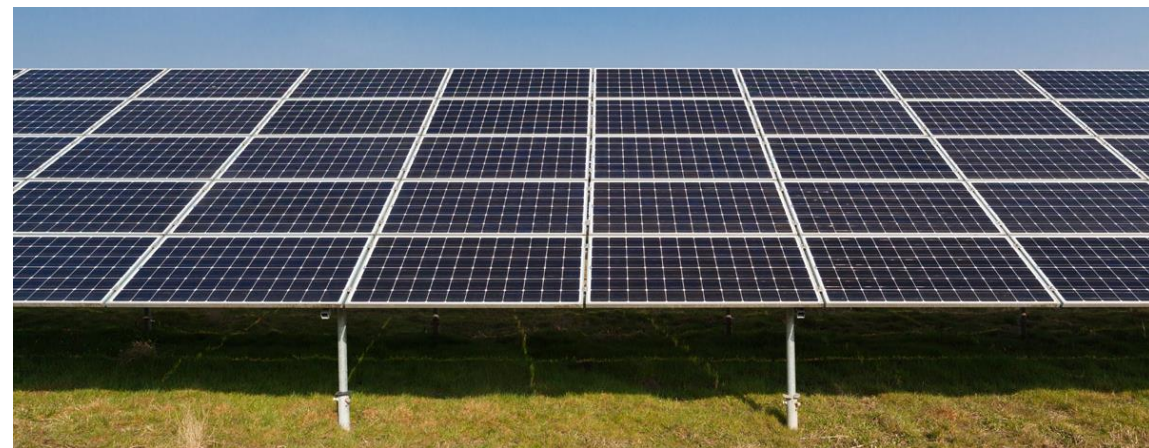
Fixed-tilt installation
