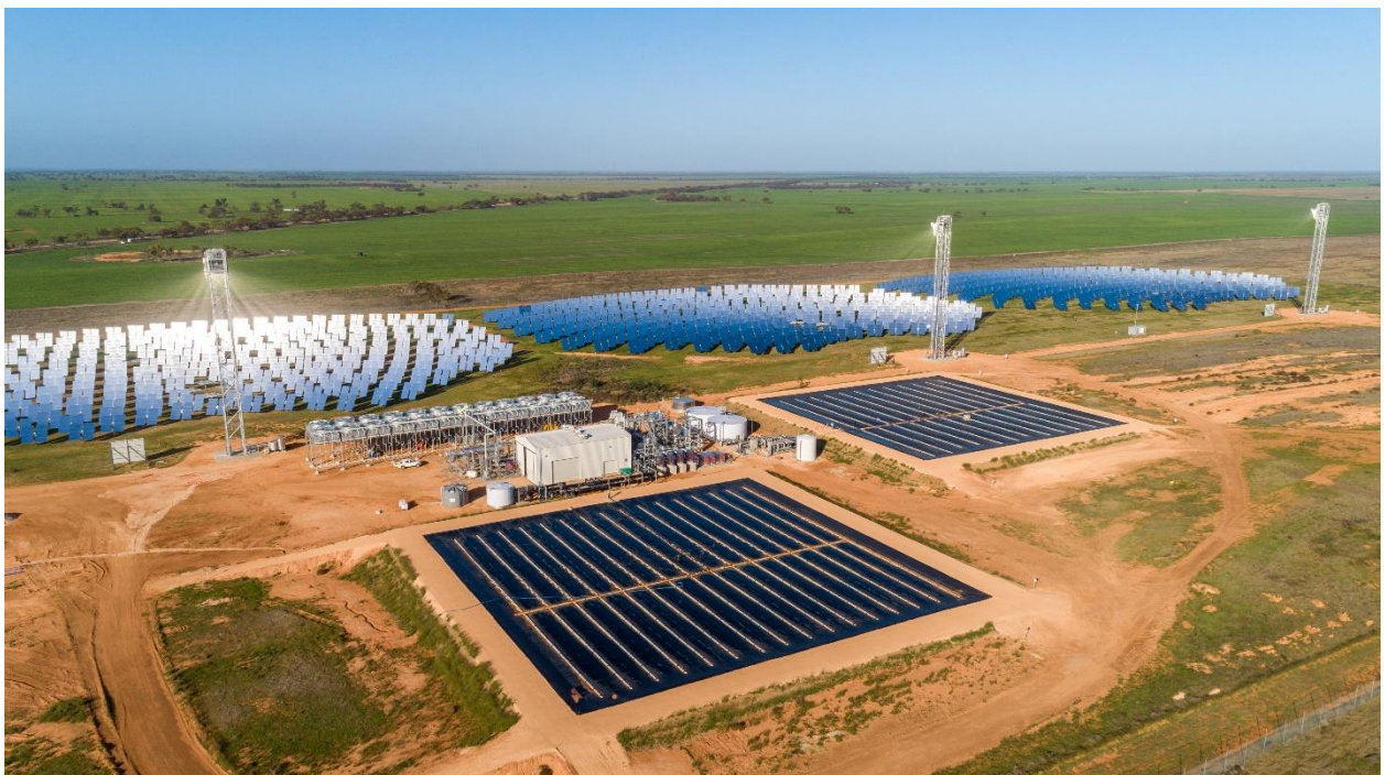
RayGen Carwarp Power Plant storage pits | © RayGen
